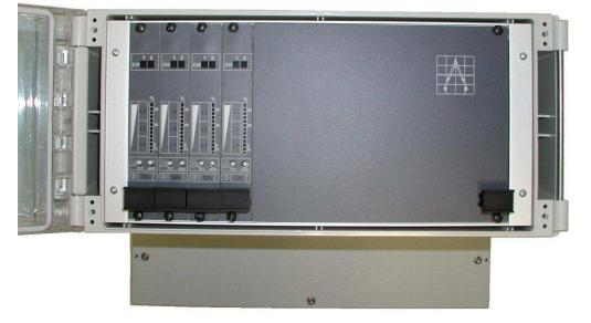
**AR400** systems are particularly suitable for small areas or on large sites, where it is preferable to have a number of small self-contained monitoring systems connected by a field bus to a remote Host system.
